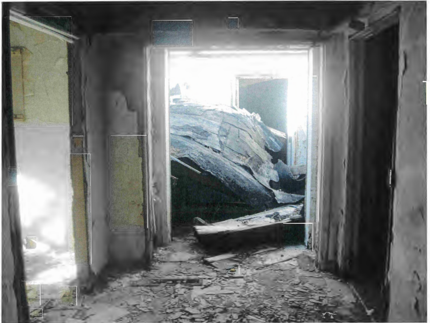
Photo 14– View of collapsed ceiling/second floor assembly into the ground floor of 110 W. Main Street. Structural collapse/compromise is evident in this location.
