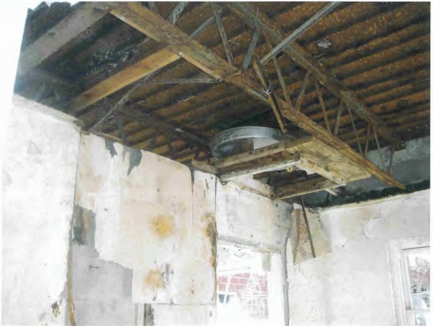
Photo 28 – Damaged/deteriorating room ceiling.
