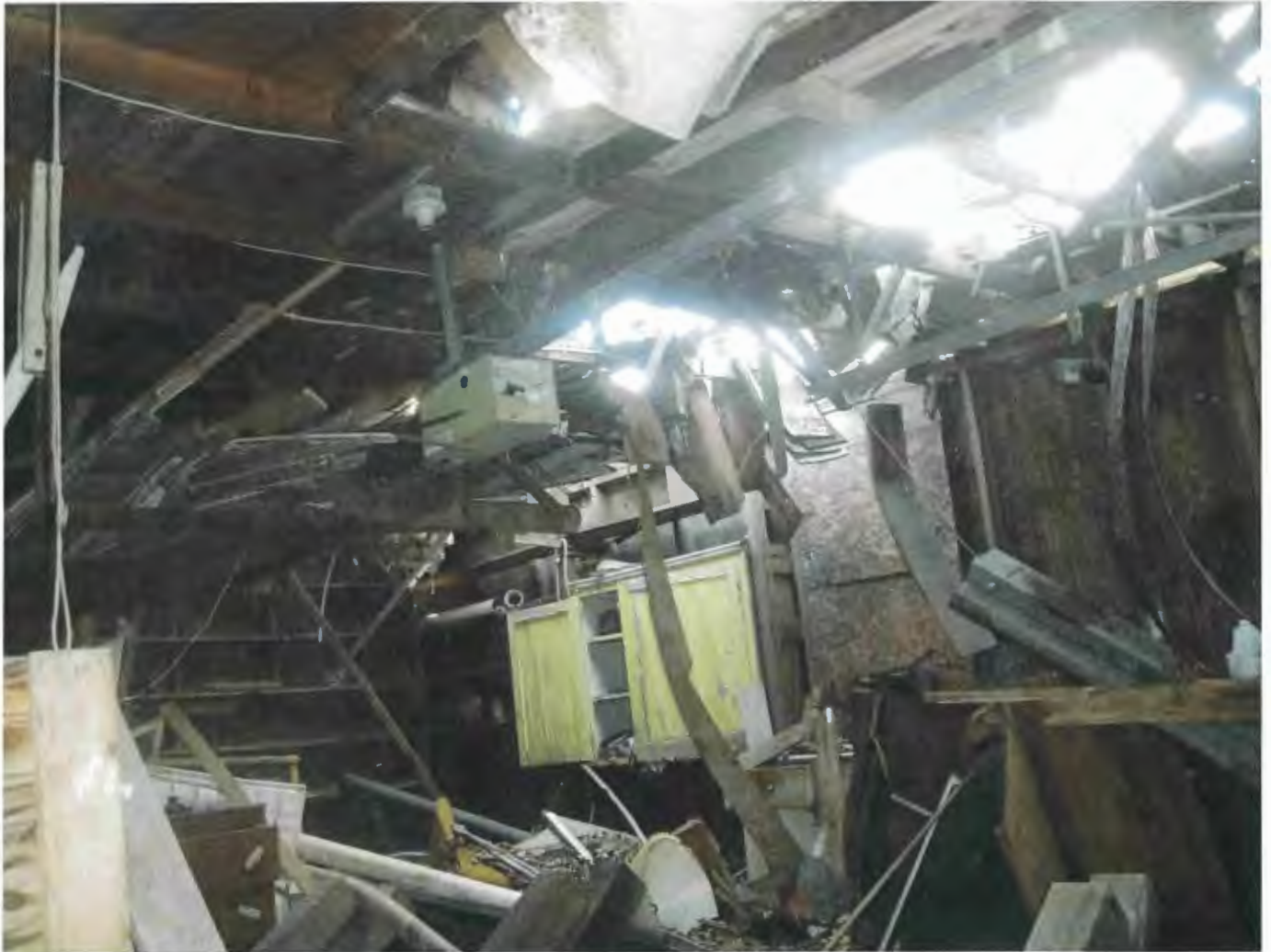
Photo 13 – View of collapsed garage ceiling.
