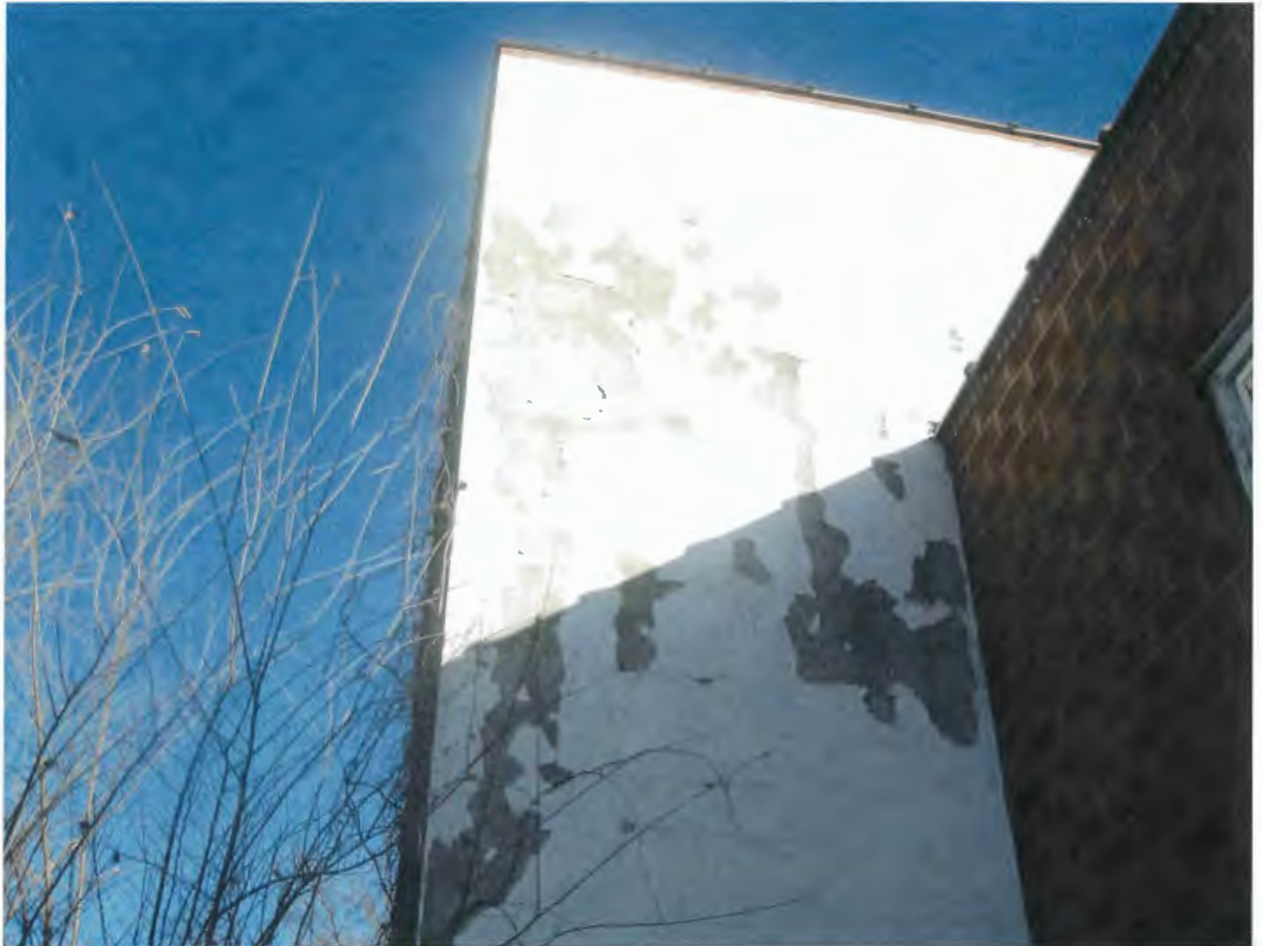
Photo 25 – Deteriorated siding material, 110 W. Main Street.
