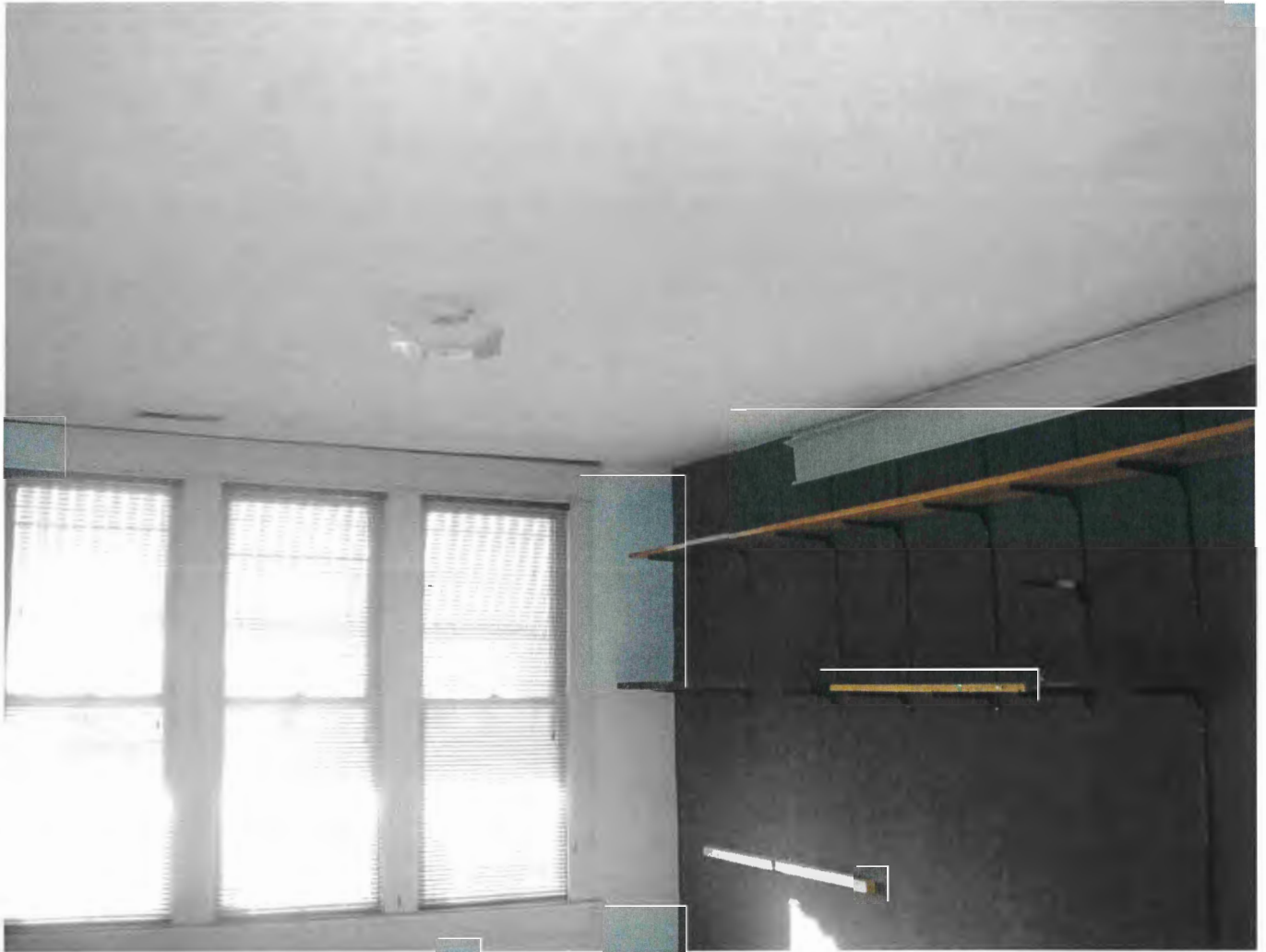
Photo 21 – Suspected asbestos containing ceiling treatment located throughout 108 W. Main Street.
