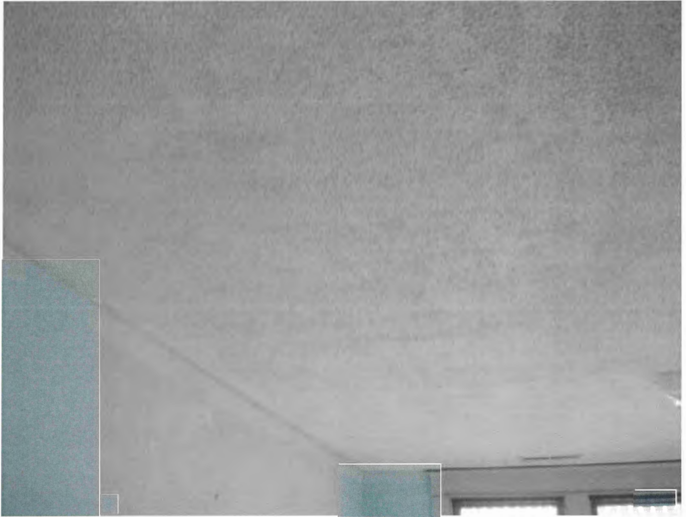
Photo 20 – Suspected asbestos containing ceiling treatment located throughout 108 W. Main Street.
